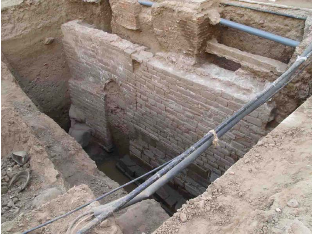
Fig. 28: Area 52: The western face of the embankment wall.
