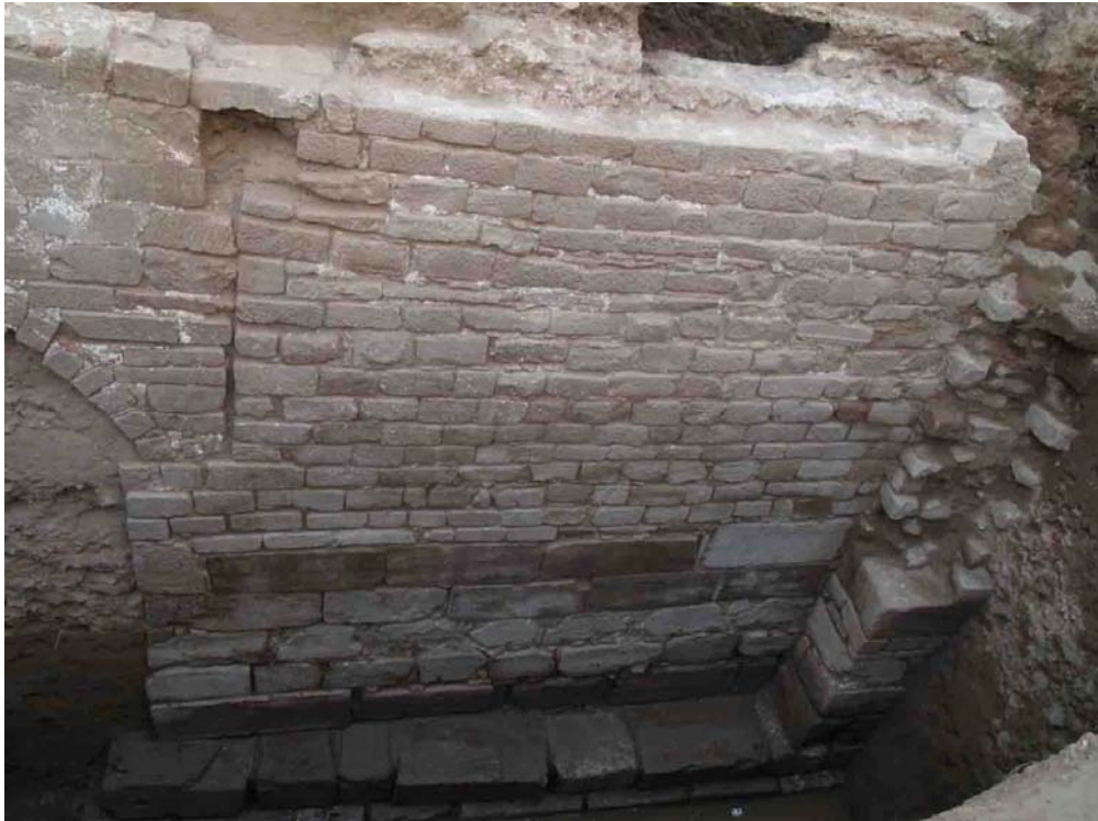
Fig. 29: Area 52: The northern part of the embankment wall.
